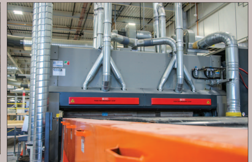
To finish, panels are sanded using a Costa to remove 1 mm from the top and bottom.
