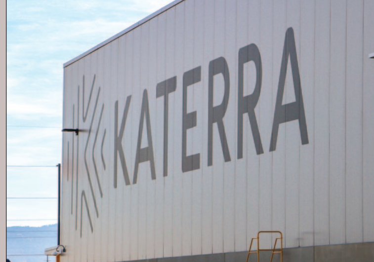
The $150 million facility's equipment was mostly supplied by USNR.
